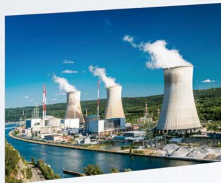
Electric power/ Power generation equipment
