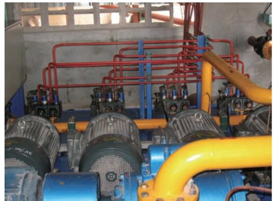
Application on monitoring lubricating oil in main pipe of main mill lubrication station in cement industry
